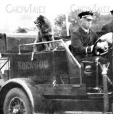
RESTORATION - 1929 Chow in Fire Engine at Saranac ...
